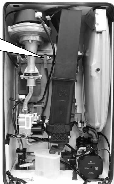
Flame Detection Electrode
